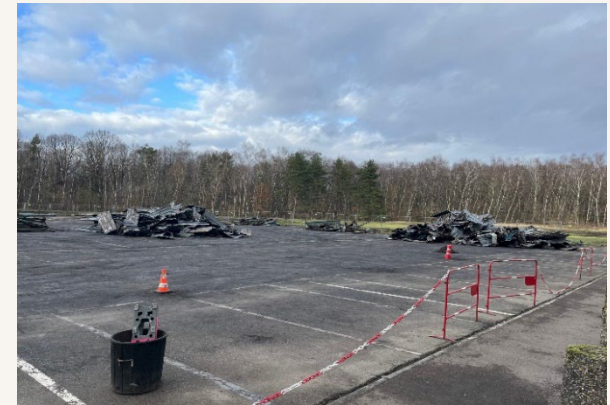
Gazel / Circa agreed site clearing underway
