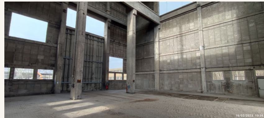
Inside Decuvage building
