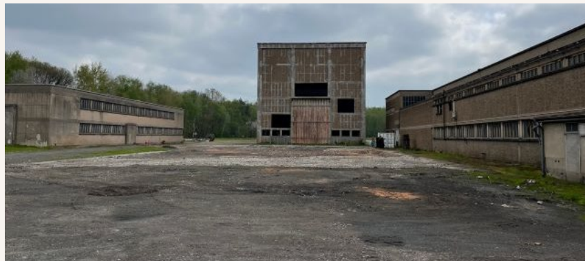
Remaining existing buildings
