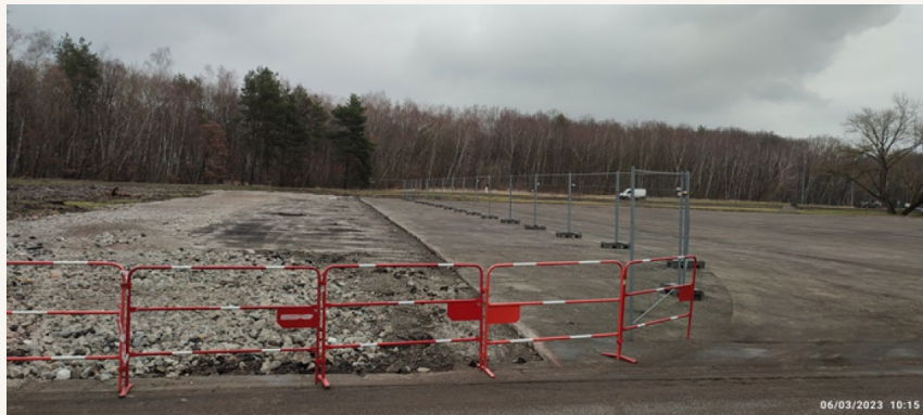
Demolished parking lot with view to woodyard area
