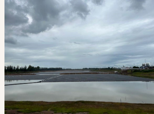
Section of the solar power plant at 304 Industrial Park in Prachinburi
