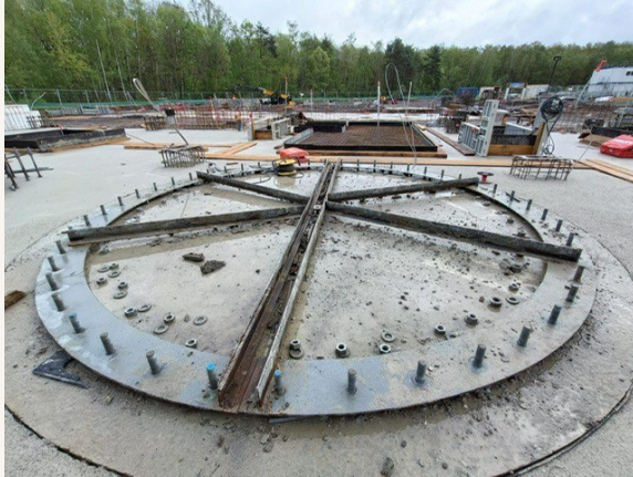
Foundation and steel frame for boiler installation
