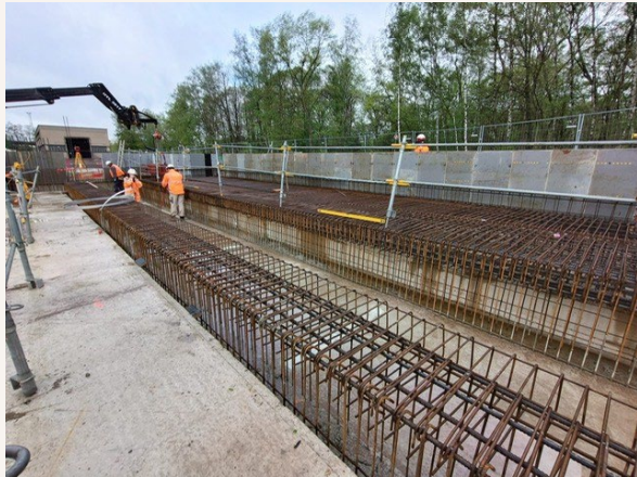
Moving floor foundation
