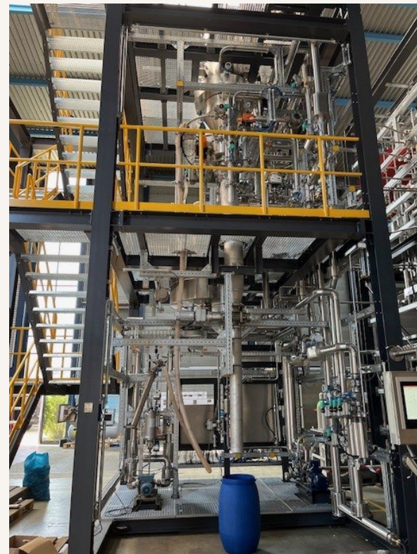
Filtration and catalyst loading
