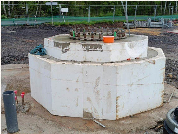
Foundation and steel frame for stack installation
